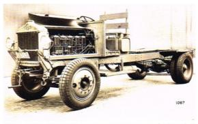
Although AEC developed its own diesel engines, a Gardner five-cylinder 5L2 found its way into an AEC in 1936.
